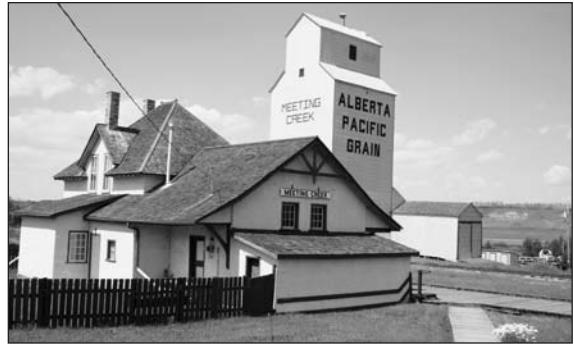
Meeting Creek Station, Grounds and Elevator.
