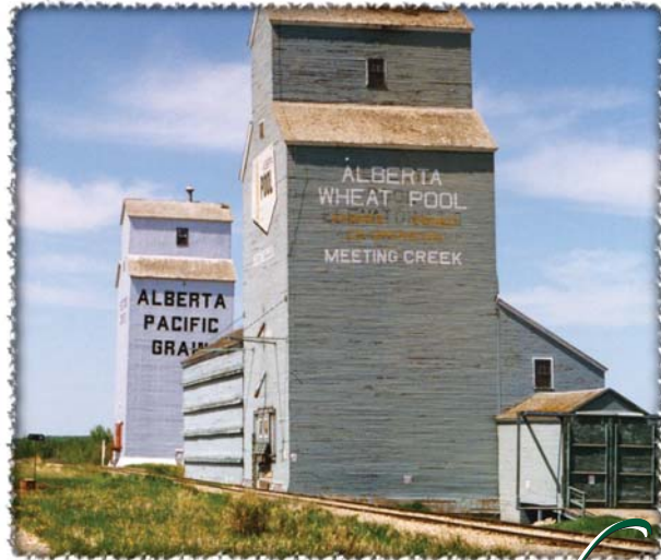
Meeting Creek elevators before restoration work started, 1987.
