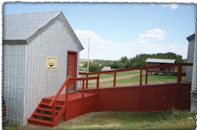
Thanks to the talents of our contractor, Graham Chillingworth, the walkway at the Meeting Creek elevator is virtually complete. The society is now searching for enough specialized tin siding to sheath the lower portion with. It looks excellent and will add greatly to the elevator. Summer, 2007.
